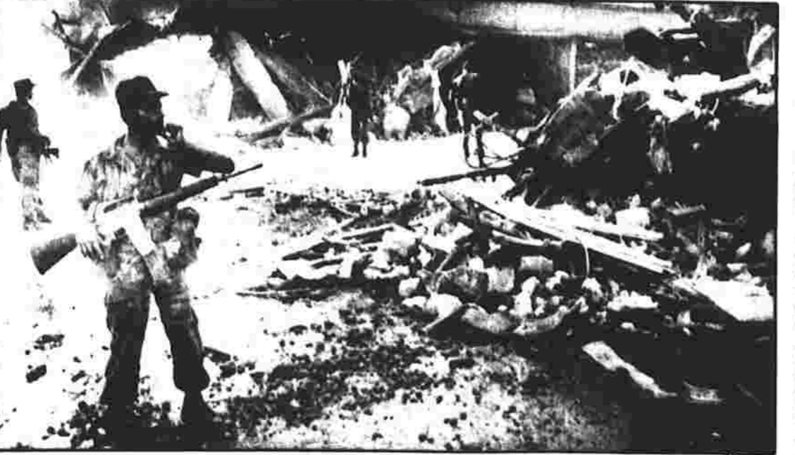
A Salvadoran soldier looks at what remains of a five-story building in the aftermath of the earthquake that struck Friday. The death toll has climbed to nearly 900.
